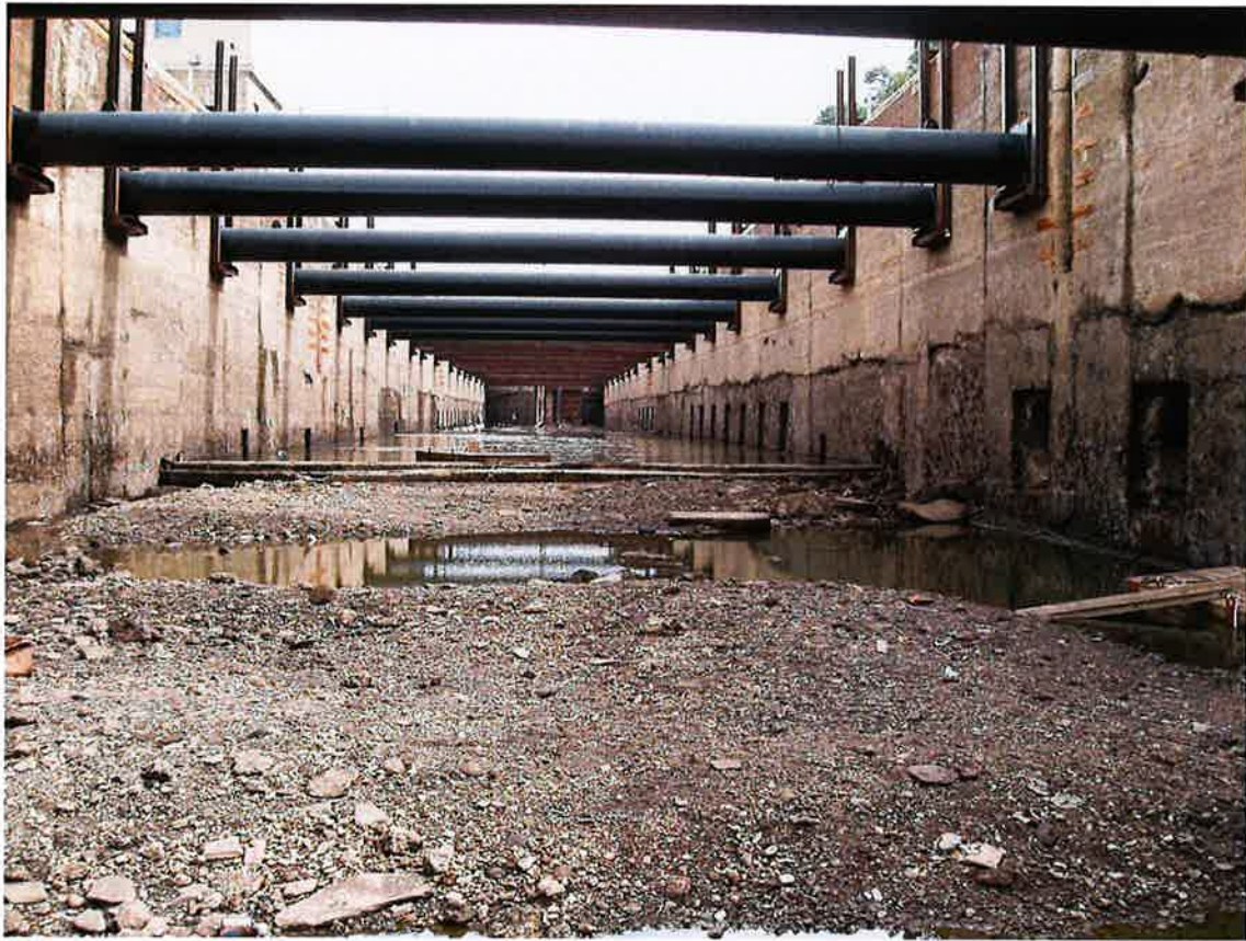
Figure 4 - Elizabeth Lock dewatered revealing its deteriorated condition
